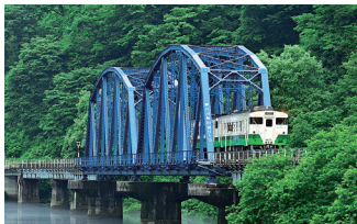
06 第八只見川橋梁 No. 8 Tadami River Bridge
