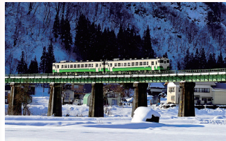
03 叶津川橋梁 Kanozu River Bridge
