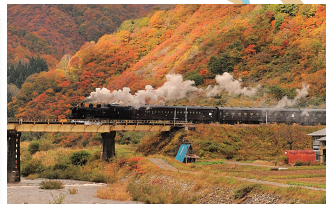
04 真奈川橋梁 Managawa Bridge
